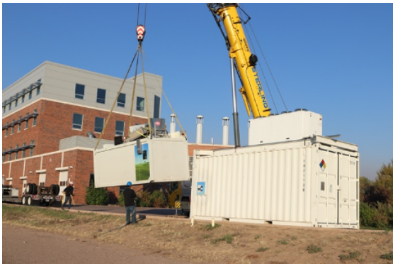
Second Container Being Lifted Into Place
